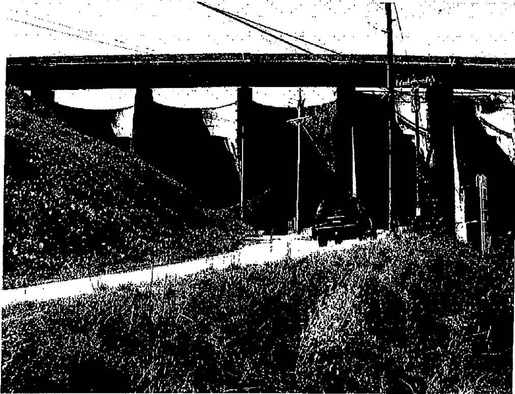
Photograph 11 Arch and Buttress Sections
